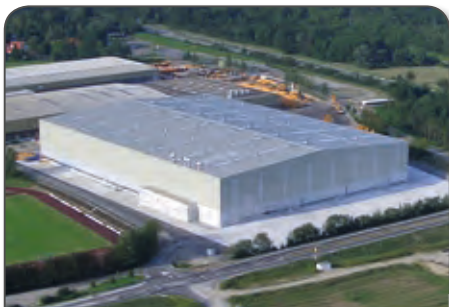
Opening of the assembly building for material handling machines
