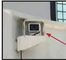
Integrated air conditioning
