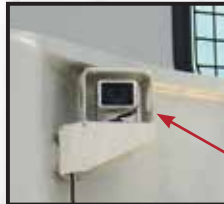
Integrated air conditioning
