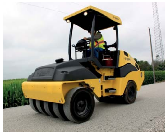
BW11RH in action on an asphalt resurfacing application
