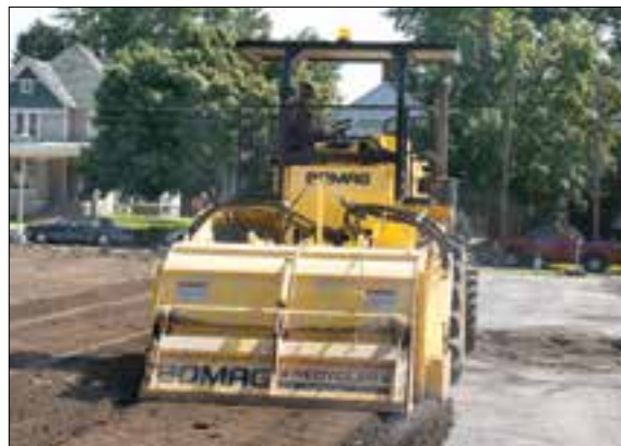
MPH362R-2 hard at work on a parking lot.
