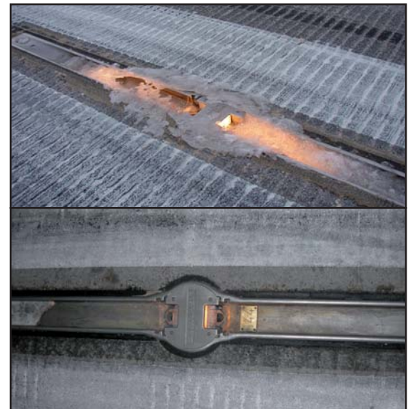
Before and after runway centerline cleaning.
