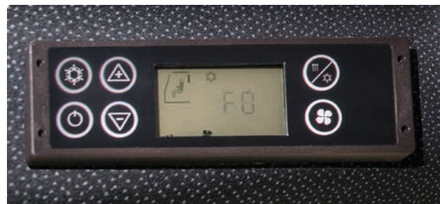
Automatic heating and air-conditioning unit control panel.
